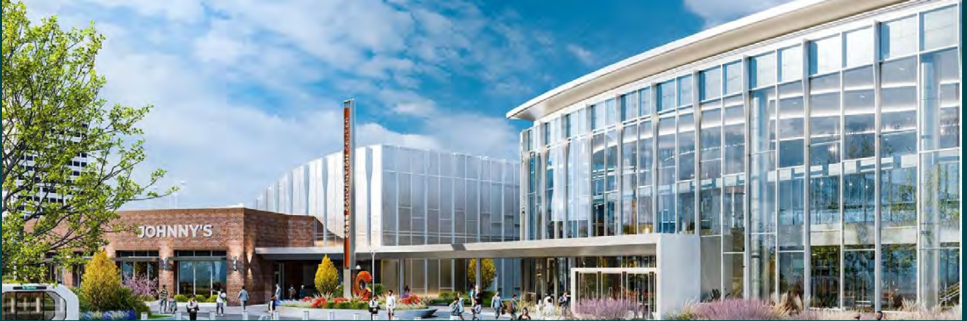
Cobb Convention Center — exterior.
